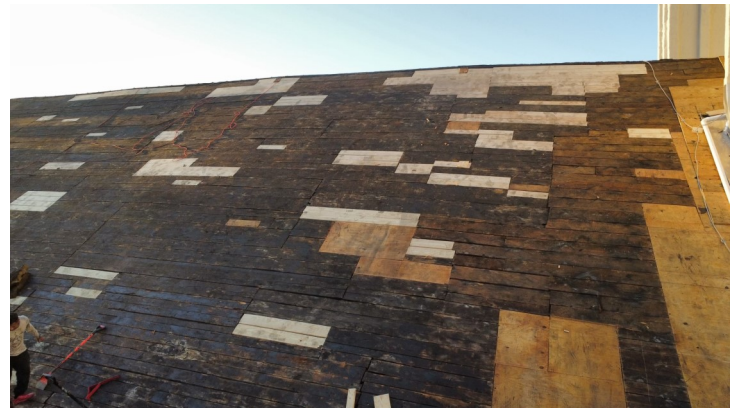
Below, all rotten lumber is removed and replaced.
