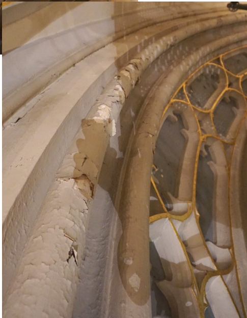
(Below) The dove at the apex of the great arch is surrounded by failing paint 52 feet above the sanctuary.
