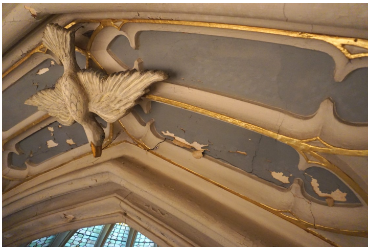
(Below) The dove at the apex of the great arch is surrounded by failing paint 52 feet above the sanctuary.
