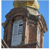
St. John the Baptist Church has endured many years with rot affecting one of the bell tower's wooden louvers. This has caused the louvers to shift or fall out all together! The area where this occurred is very visible to the passers-by on the elevated Pontchartrain Expressway. Upon closer inspection, it appears that the damaged pieces can be replaced rather economically. Therefore, with financial help from our
